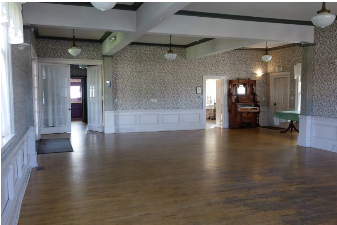
Figure 49. First floor event volume looking southeast. The event support space is at left behind the French doors and the kitchen is at right through the doorway adjacent the organ. The south doorway is at the far right below the exit sign. The light fixtures are ca. 1924, and the flooring and French doors from ca. 1925-1929.
