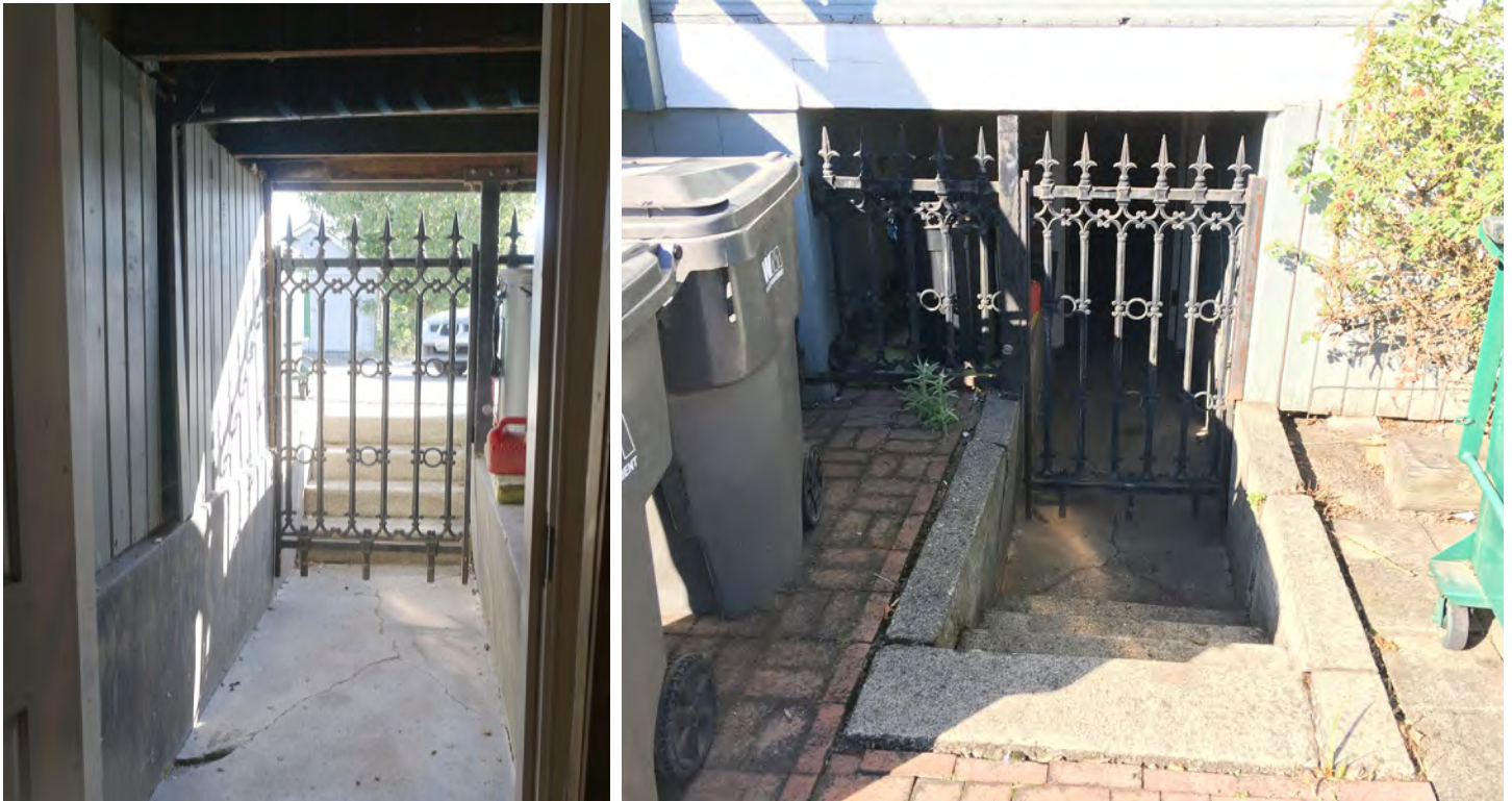
Figure 40. Rear basement entrance looking from the basement out (above left) and from the exterior down (above right).
