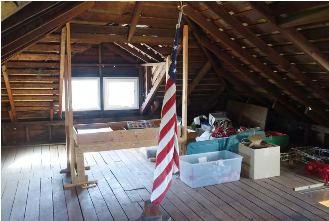
Figure 70. Attic looking east.
