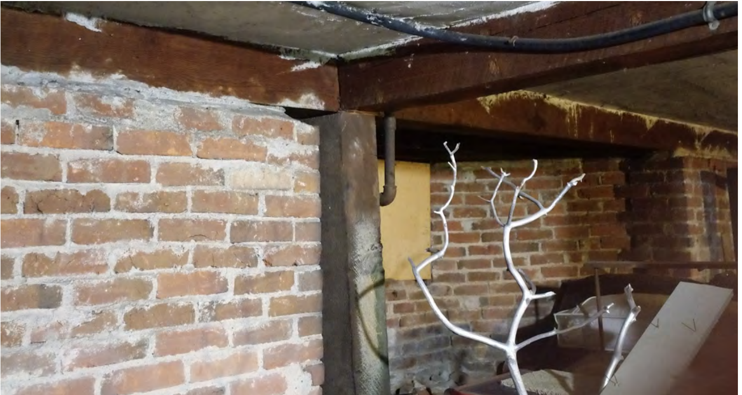
Figure 46. Basement looking northwest towards the canted portion formerly below the front bay.
