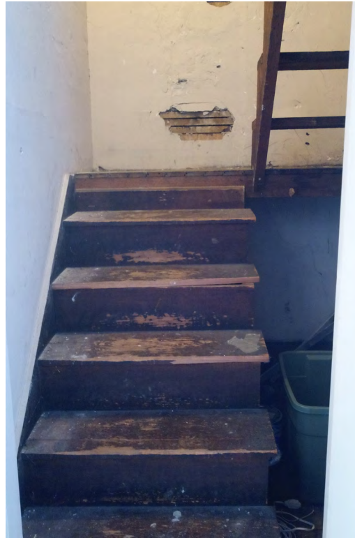
Figure 68. Stairwell within the small second floor room leading up to the attic.
