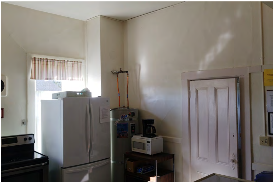
Figure 57. Kitchen looking southwest.
