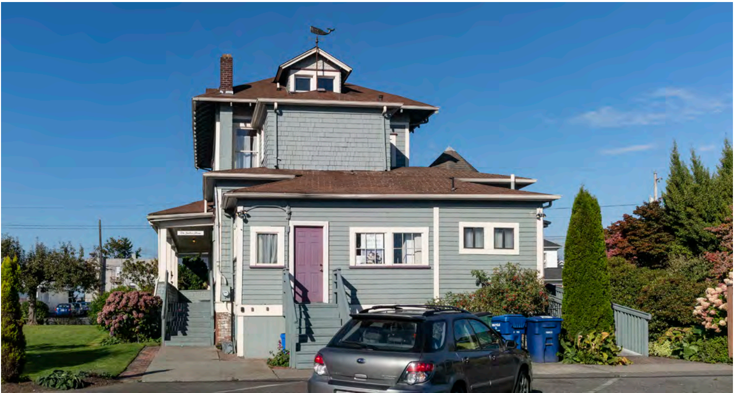
Figure 22. Rear east facade.
