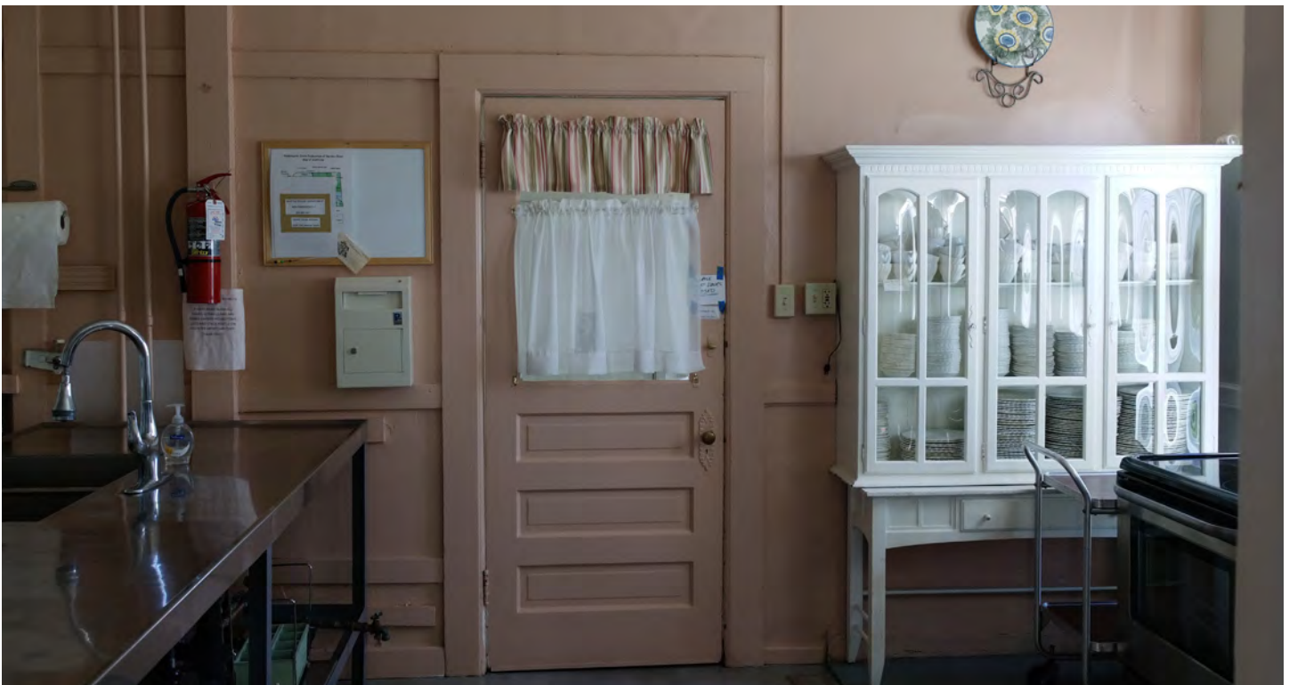
Figure 55. Kitchen looking east towards the east porch addition (lower) and a detail of the scored plaster wainscot in the kitchen (upper right).
