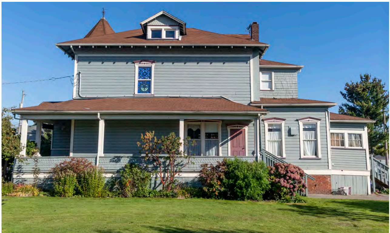
Figure 23. South side facade.
