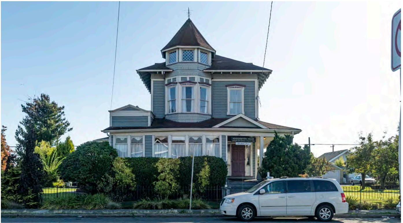
Figure 18. West front facade.
