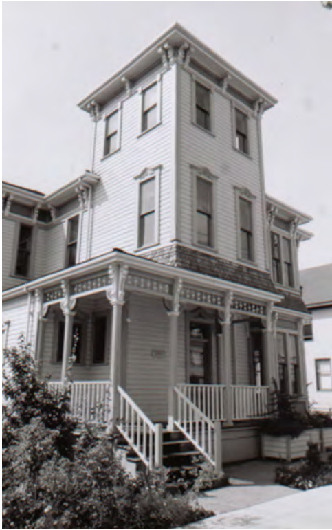
Figure 78. George W. Ward Residence (1882). Courtesy Department of Neighborhoods, Historic Resources Database.
