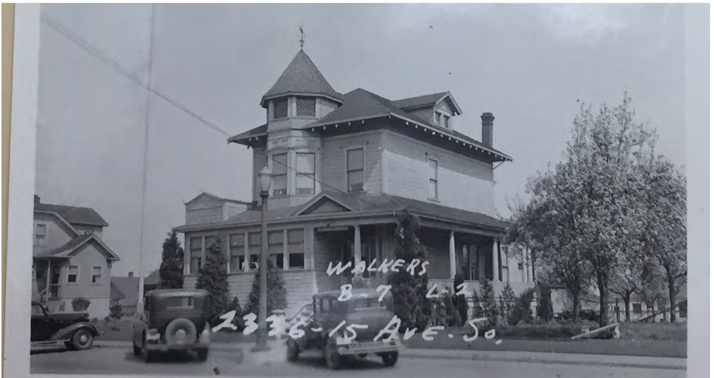
Figure 75. Ca. 1937 view of the house. Source: Puget Sound Regional Archives, property record card.
