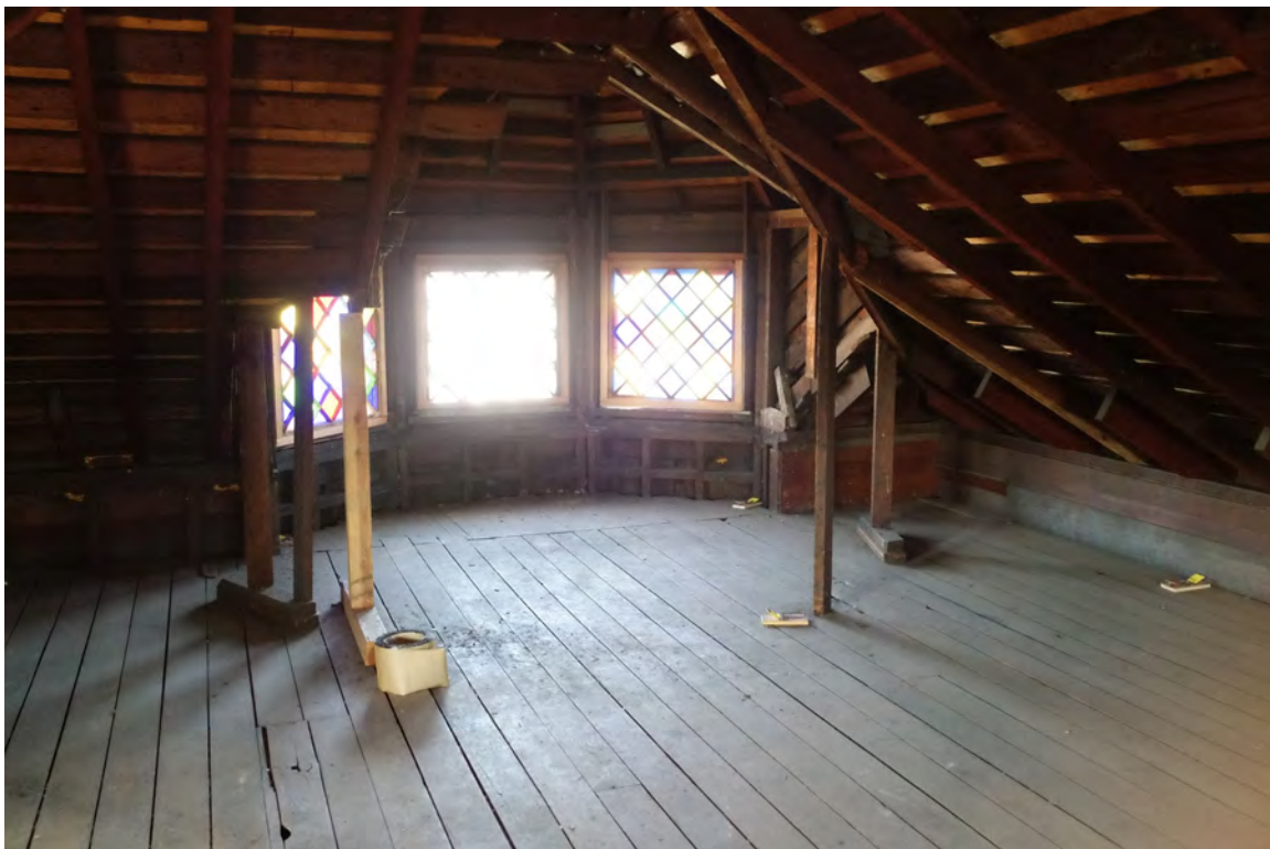
Figure 69. Attic looking west into the front bay with the stained glass windows.
