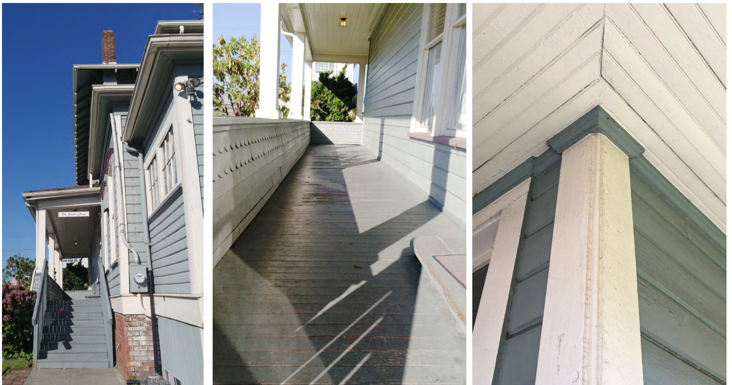
Figure 41. South porch, east stairway (above left), south porch looking west (above center), and corner detailing at the south porch on the southwest corner (above right).
