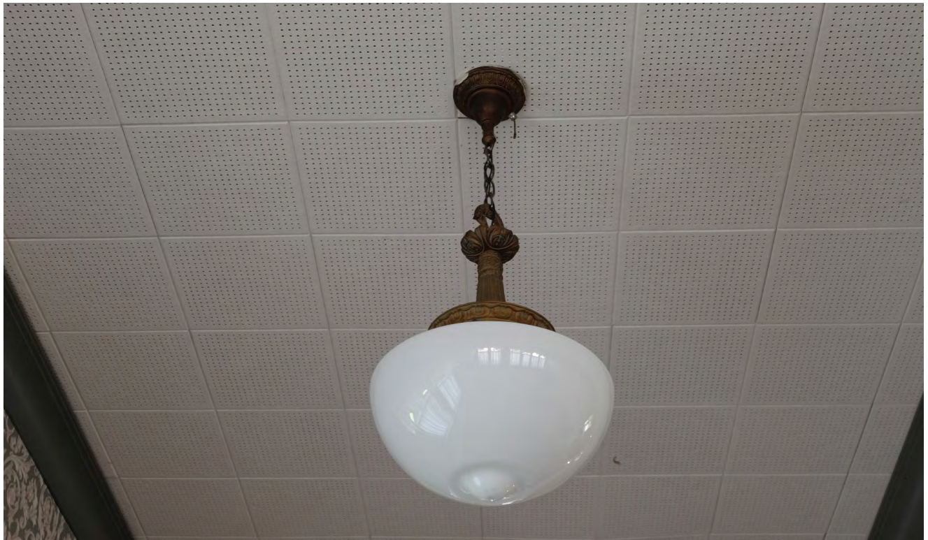
Figure 52. Light fixture detail, ca. 1924.
