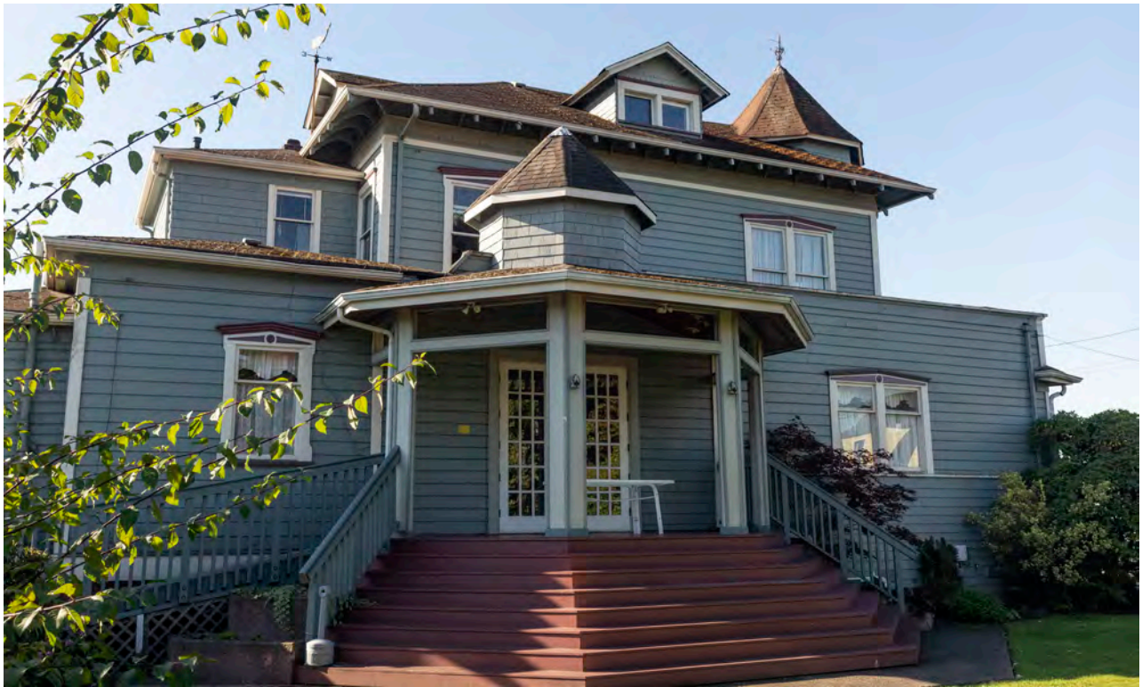
Figure 20. North facade looking southwest.
