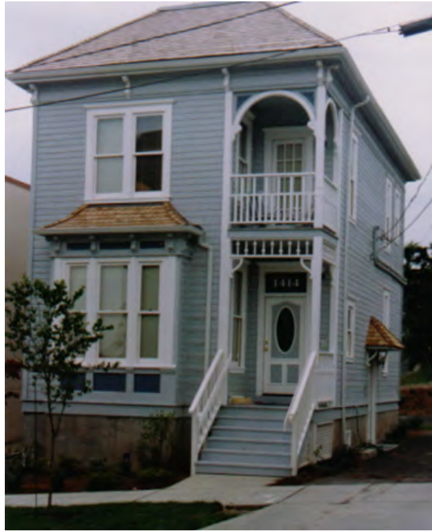
Figure 79. 1414 S Washington Street residence (1901). Courtesy Department of Neighborhoods, Historic Resources Database.
